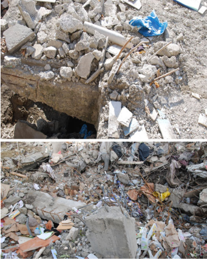
Fig. 2 Views of the collapsed building after Van earthquake
