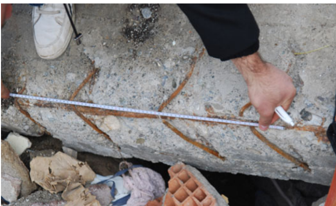
Fig. 3 View of transverse reinforcement of the building
