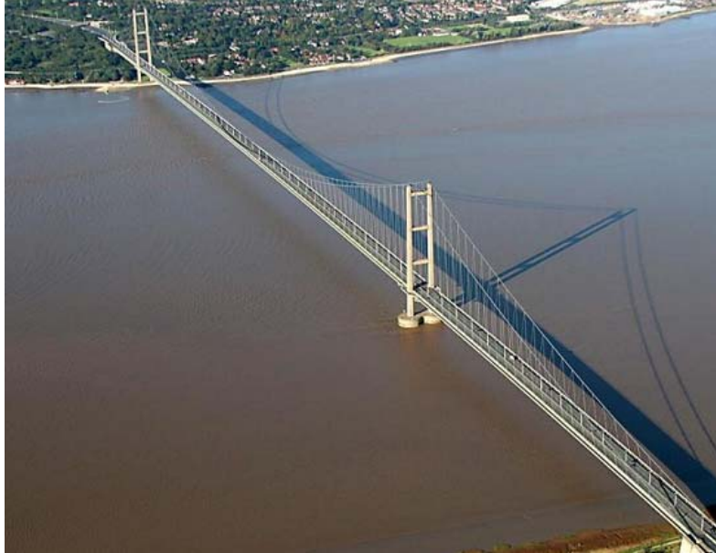
Fig. 11 View of Humber Suspension Bridge
