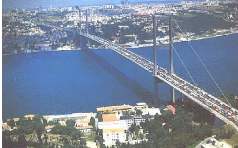
Fig. 6 View of Bosphorus Suspension Bridge
