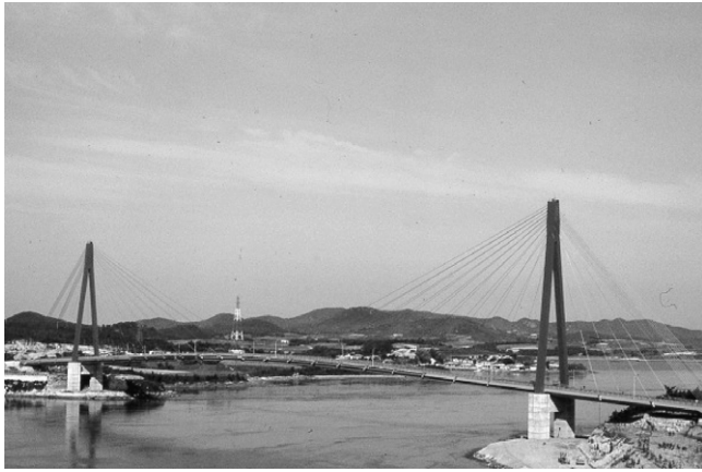
Fig. 1. Jindo cable-stayed bridge.
